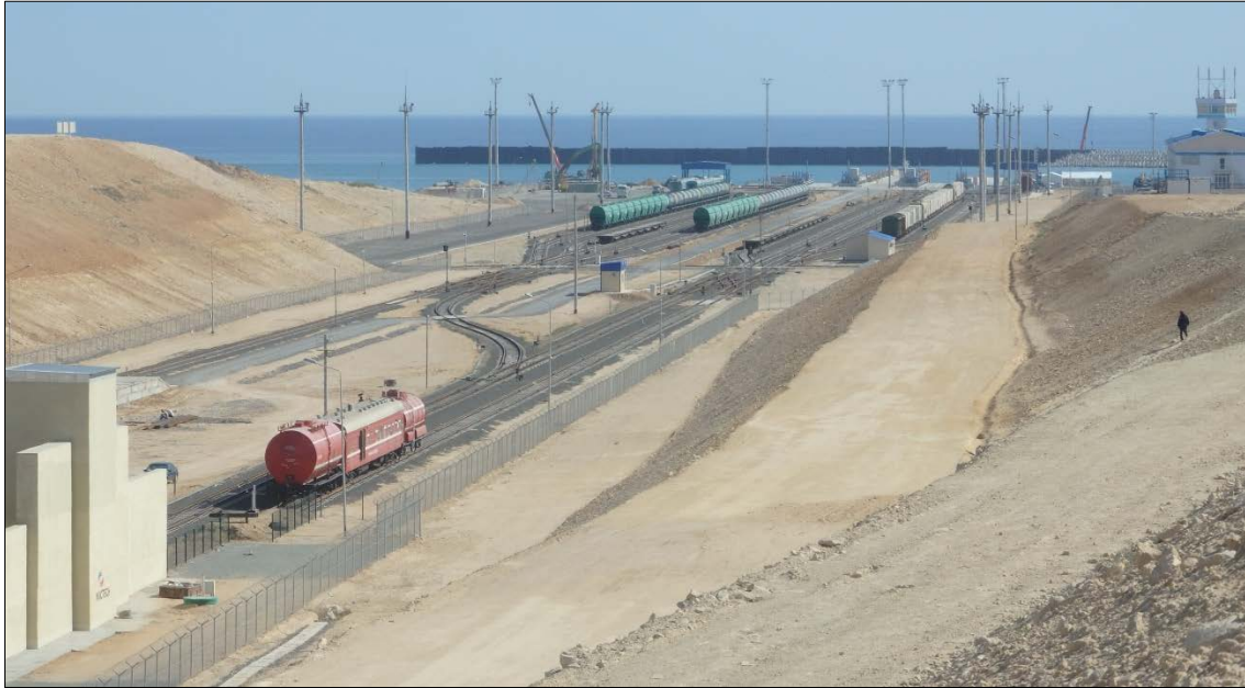
Figure 2: Ferry Terminal at the Kuryk Port
