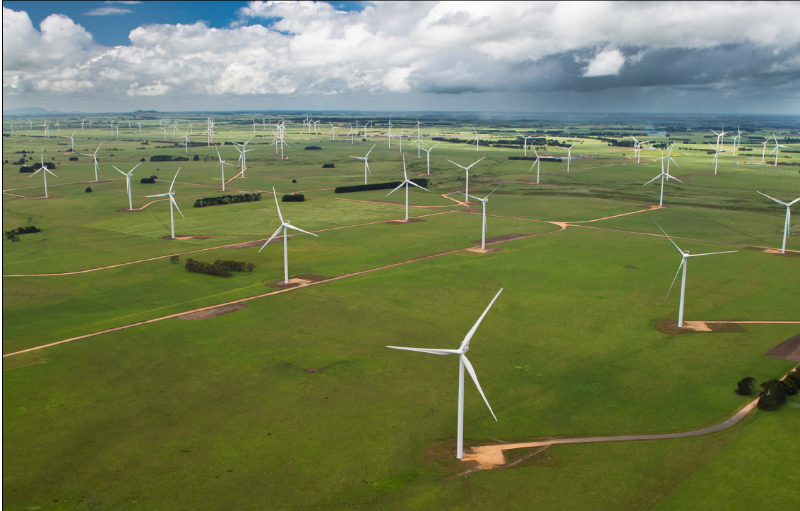
Figure 1: Horizontal Axis Wind Turbines (HAWTs)
