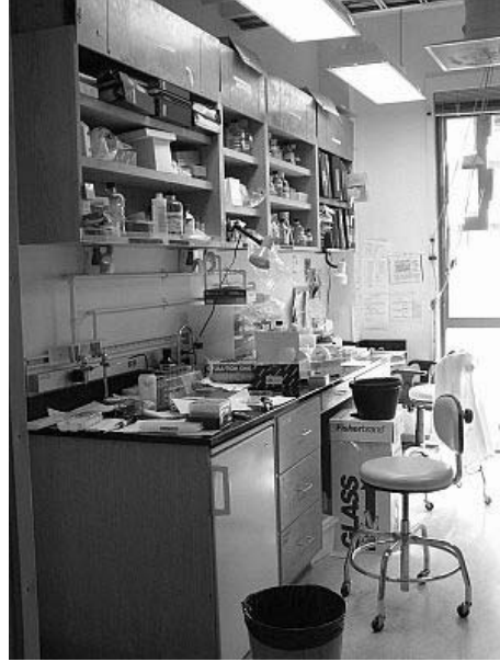
Figure B.10: Shelves with metal restraints (top)
