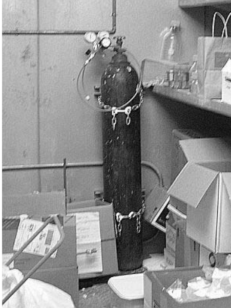
Figure B.5: Smaller tank restraint
