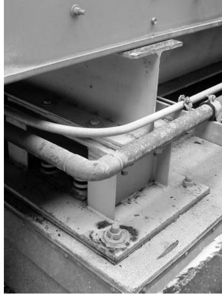
Figure A.4: Chiller support
