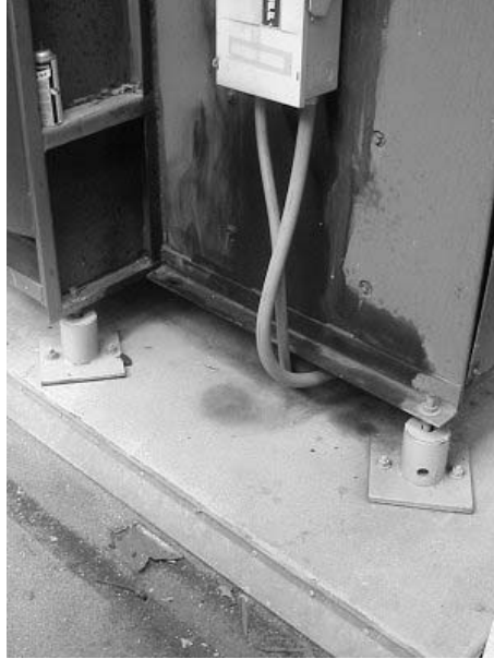
Figure A.3: Rooftop cabinet support
