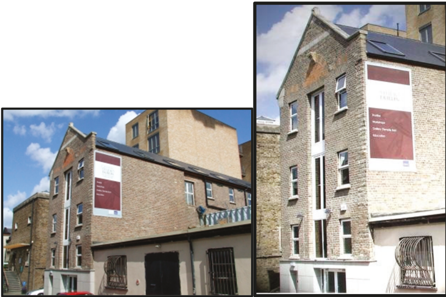
Figure 5. The four-storey converted granary, new printmaking studio for GSD.
