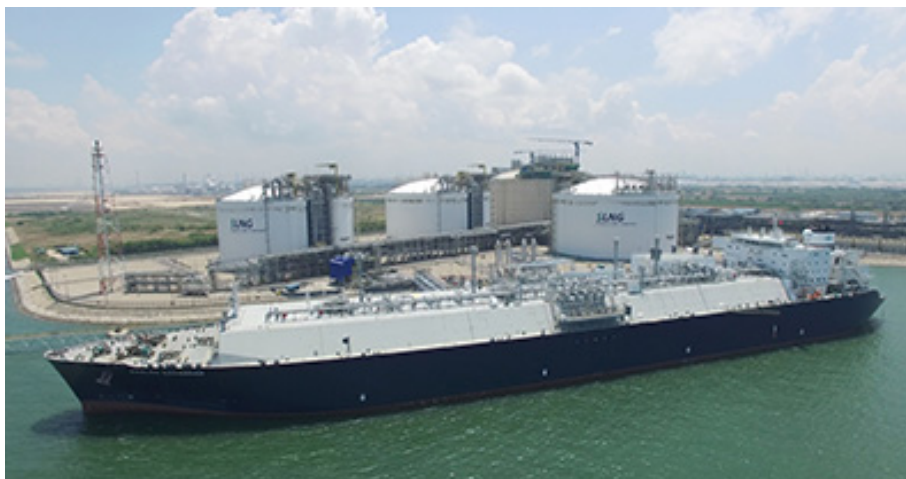
Figure 9: Singapore LNG (SLNG) regasification facilities
