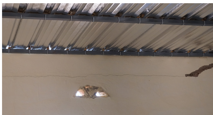
Cracks in the wall of a newly constructed house for resettlement in the new Bouly village (Photo: Merle Groneweg, 2017)
