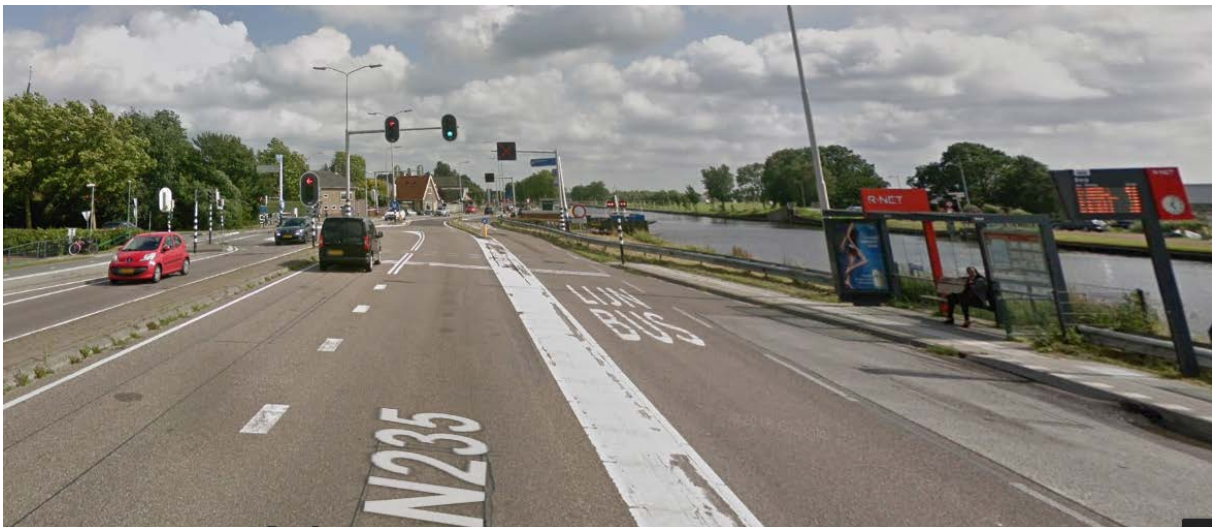
Figure 7: Image retrieved from Google maps (July 2016) to illustrate the safety situation at Ilpendam.
