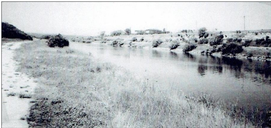
Figure 5. Drainage channel in Iași county, non-lined (2009) (Author's archive)
