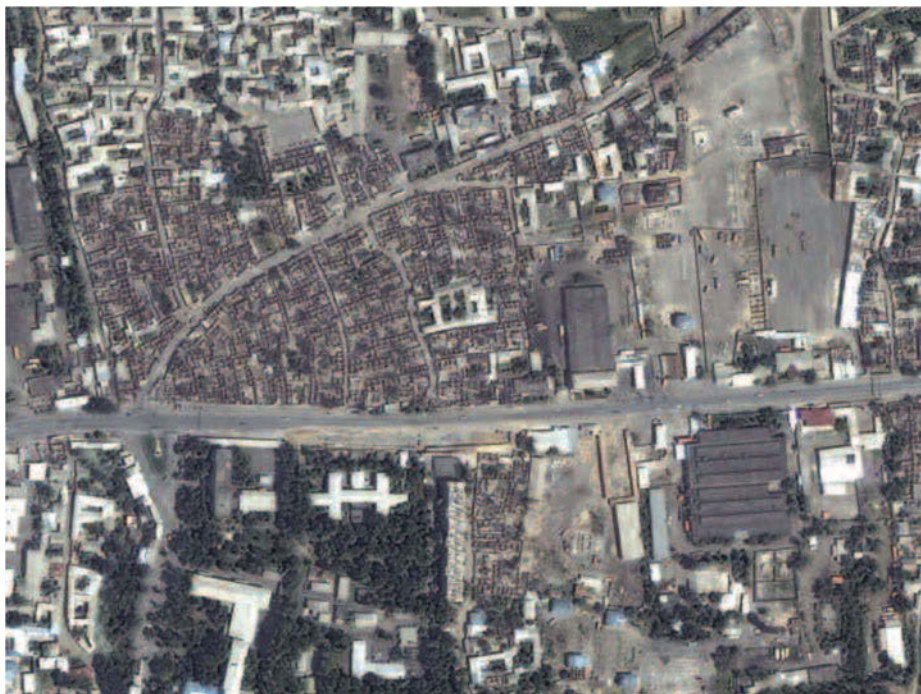
FIGURE 3. Destruction During the 2010 Osh Riot (Detail)
