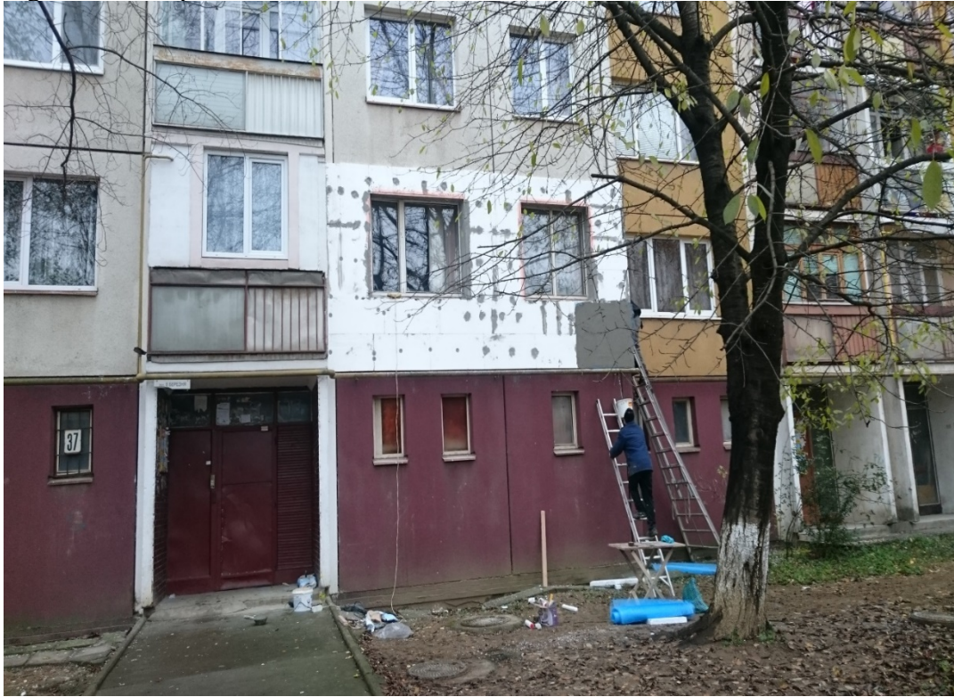
Figure 3. Example of visible EE renovations (addition of wall insulation) in Uzhhorod.
