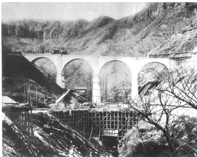
Figure 8: Construction Work in Steeper Areas (The Usui Pass)
