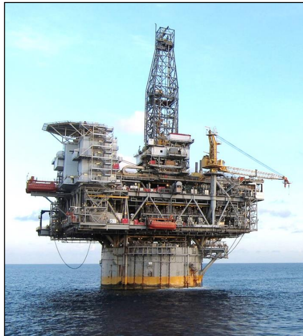
Figure 4. Example of a Platform Rig: The Mad Dog Spar in Deep Water in the Gulf of Mexico
