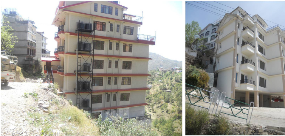
Fig. 12. Multistoried buildings with partial basements in Sector III, New Shimla Township.
