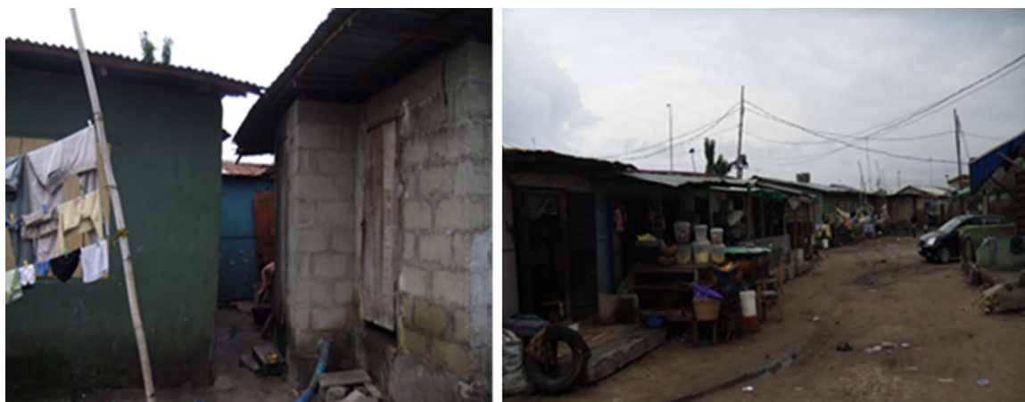
Fig. 5. Infrastructure and building conditions at Ikeja and Eti-Osa.
