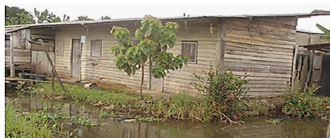
Fig. 2. Temporary structure erected with wood (Carabotte).
