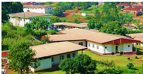
Fig. 3. Standard structure erected with blocks.
