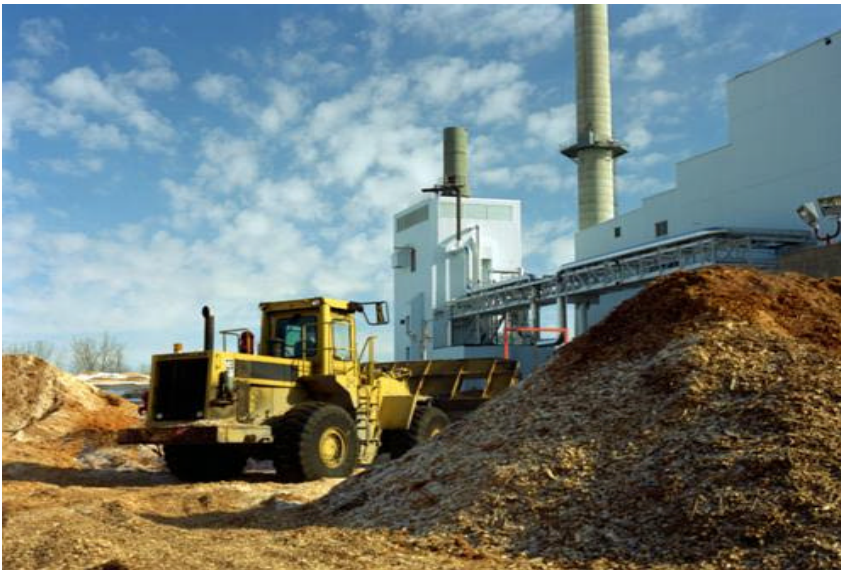
Photo 3: Modern biomass power plant
