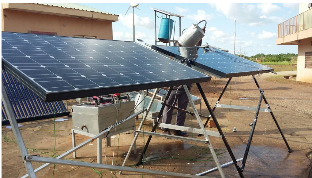
Fig. 6. Manual water spraying of the module.
