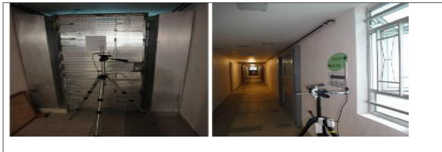
Fig IEQR3 Checking ventilation device
