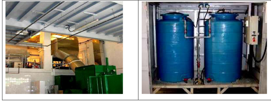
Fig IEQR2 De-odorizes at the Covered Refuse Collection Points
