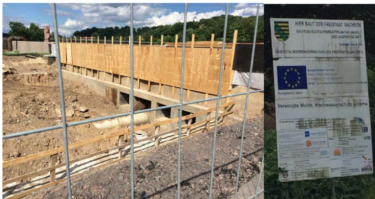
Figure 31 Floodwall, project 4, under construction (June 2017).
