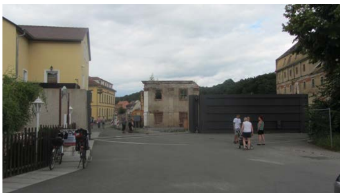
Figure 27 Floodgate, part of the floodwall Project 1.
