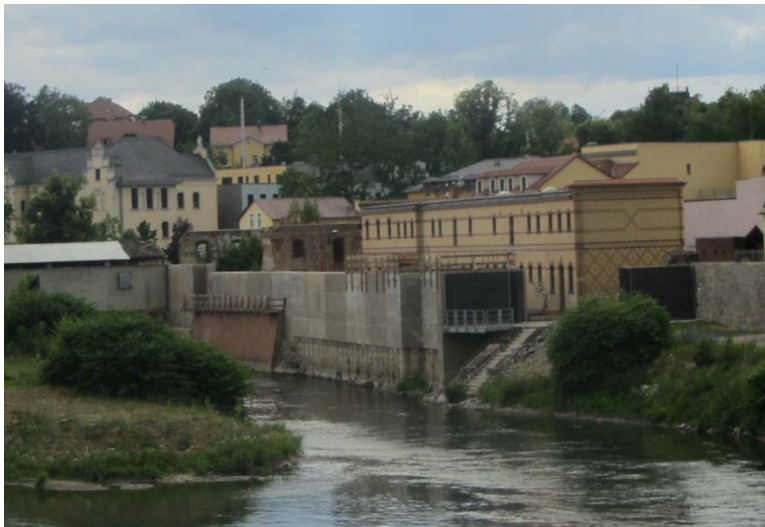
Figure 29 Floodwall, Project 2, under construction (June 2017, author).
