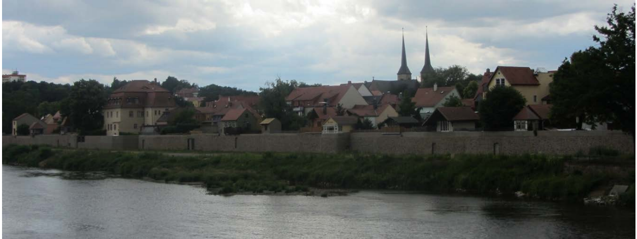
Figure 33 New floodwall, photo taken across the Mulde River by the author (June 2017).
