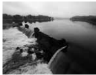
TNC: Integrated Reservoir Floodplain Management, Georgia and South Carolina, USA
