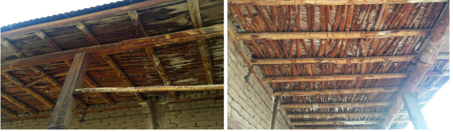
Figure 10. The Supporting Bonding Timbers of the Roof
