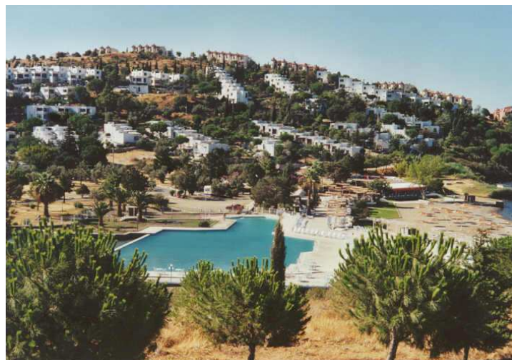
Figure 3. Residential units with deck roofs at Artur.
