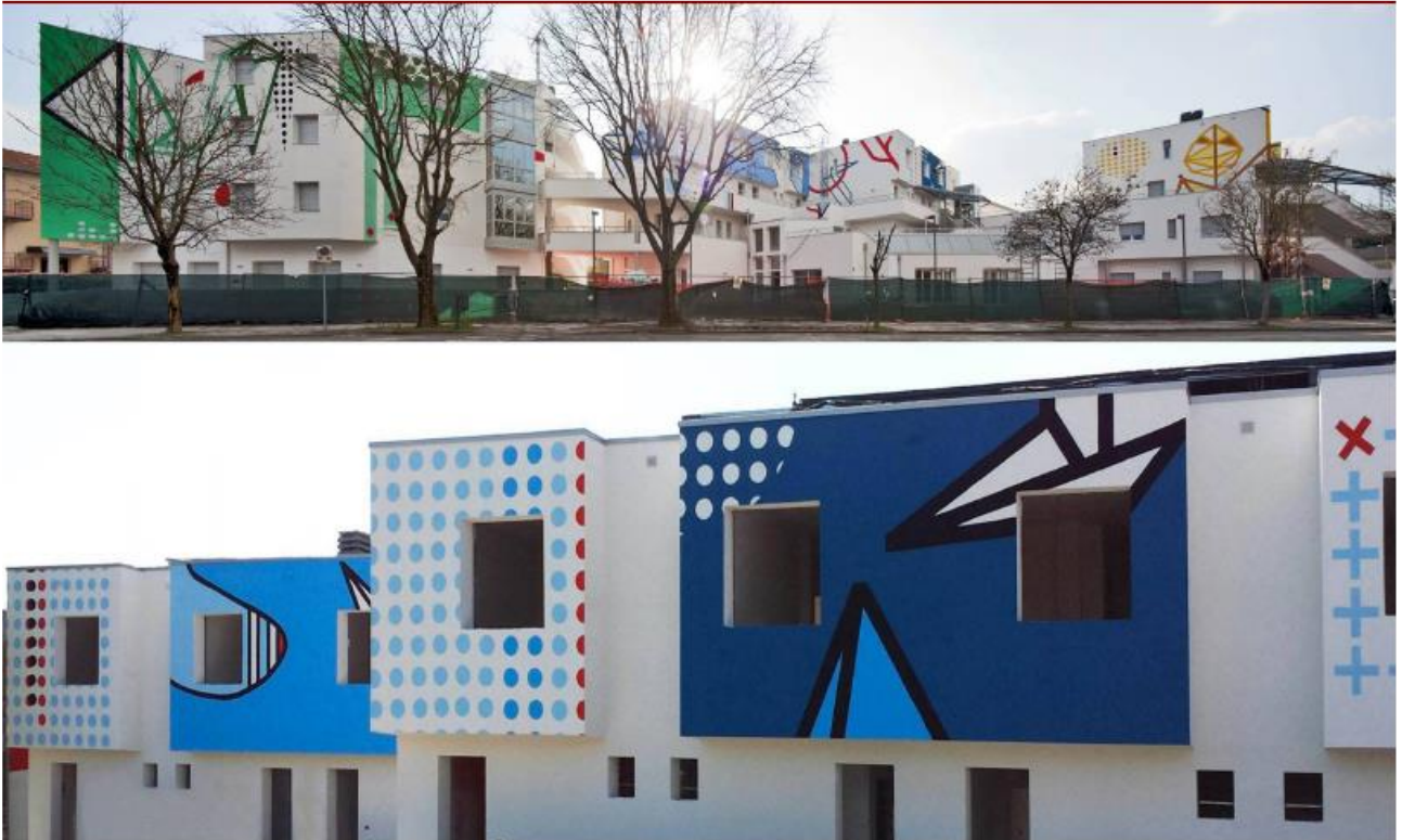
Fig. 5 How re-generate districts of social housing: with realism and participation; Faenza, Fornarina street
