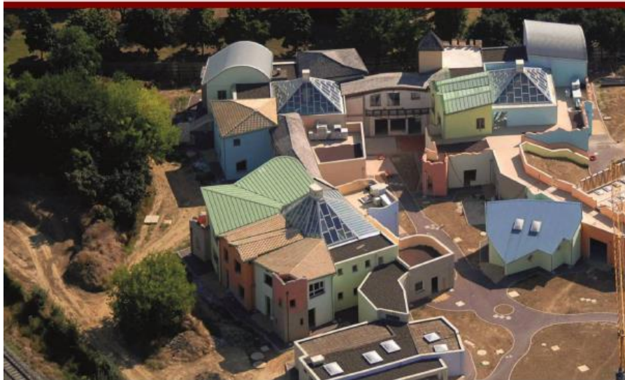
Fig.7 Public works and bio-architecture: acting with public example; Faenza, Don Milani school
