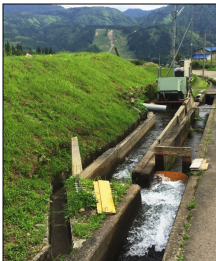
Photo 1 (left) and 2 (right): Installation examples of generator in Itoshiro, Japan
