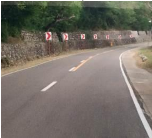
Completed Portion of the Case Study Project with installed Road Safety Devices from Phase 1
