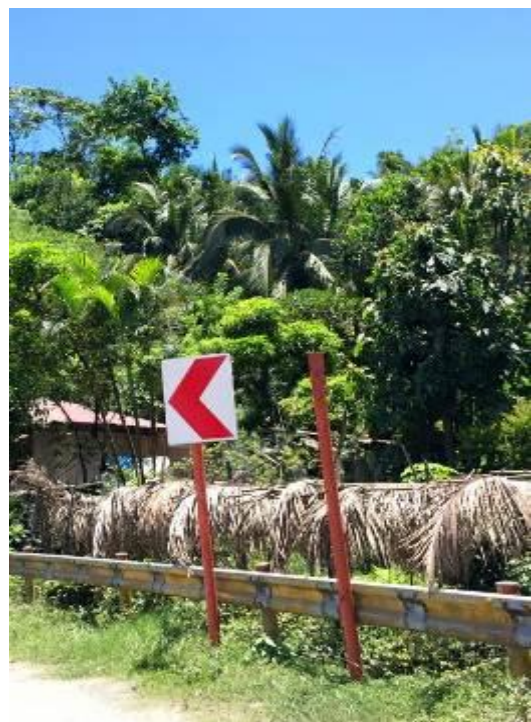
Figure 21. Poles with missing traffic signages
