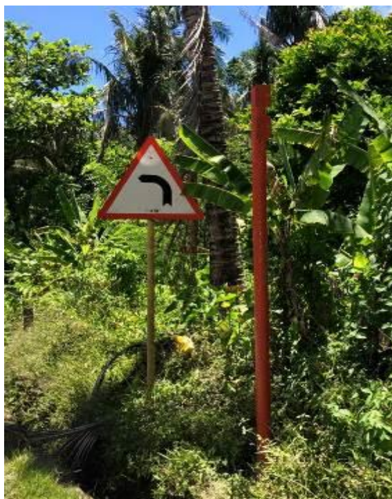
Figure 21. Poles with missing traffic signages
