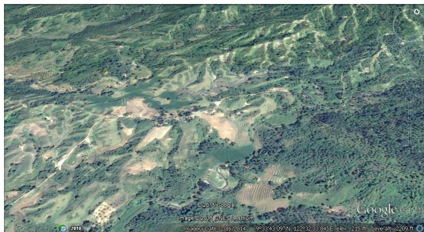
Figure 22. Eroded Areas in Hinobaan, Negros Occidental (Google Earth).
