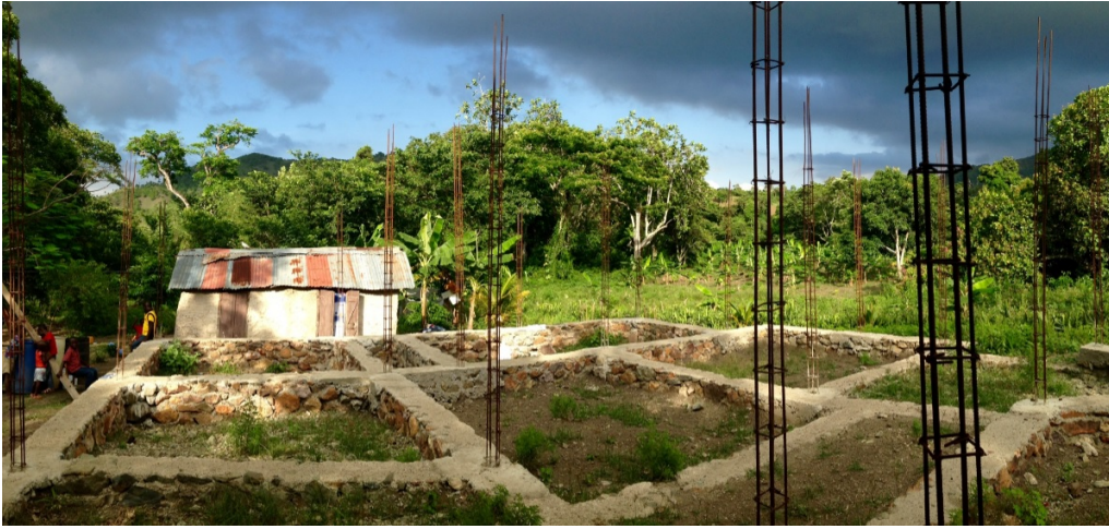
In the foreground is the foundation for the new home of a worker allowed to work in the US in 2015, under construction in 2016 for his family of seven. In the background, his current two-room home. Taken May 22, 2016 in Milot, Nord by Hannah Postel.
