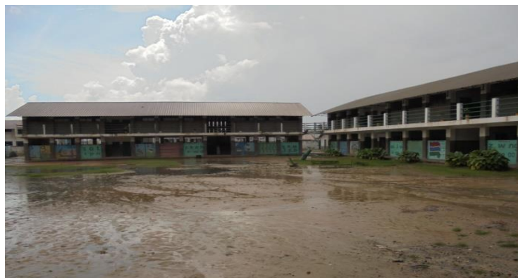
Figure 7: Inundated school compound
