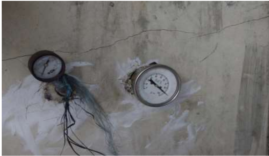
Figure 20. Pressure and temperature gauges of a flatbed dryer in Alaminos, Pangasinan. Gauges should be properly labeled and replaced as soon as possible if malfunctioning. The temperature gauge at the right is showing a temperature reading of 90oC; however, drying temperature of rice paddy is supposed to be 40-45oC. Is the gauge malfunctioning or is it measuring air exhaust of the biomass furnace directly?
