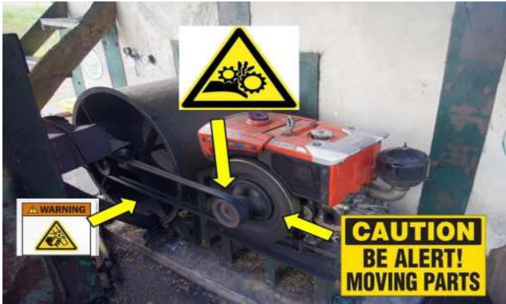
Figure 21. Some flatbed dryers need retrofitting of safety shield for rotating / moving components.
