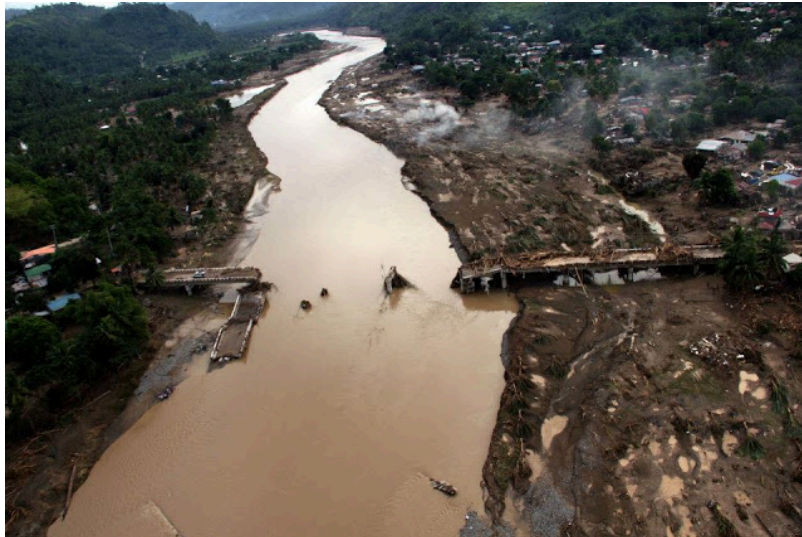
Picture IV.B.4. The old Mandulog Bridge Washed Out/Destroyed by TS Sendong
