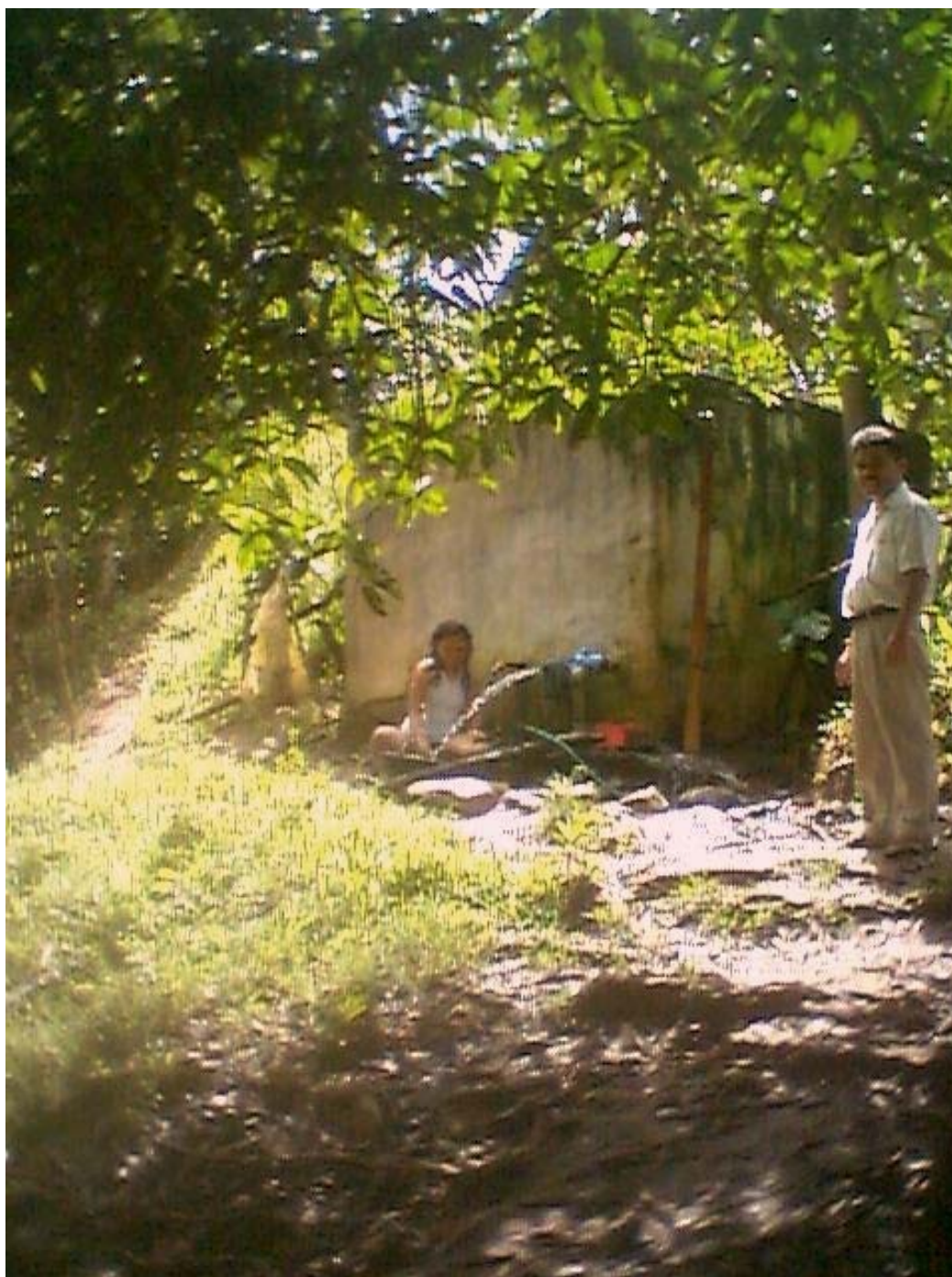
The spring box (communal water point) where the water pipes are connected. Barangay residents also get water from this source for their other household needs.
