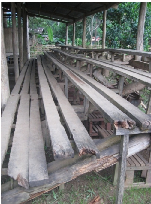
Dilapidated Multi-Purpose Hall in Afga Central Elementary School—one example of a project that could be financed through voluntary contributions by mobilizing resources.
