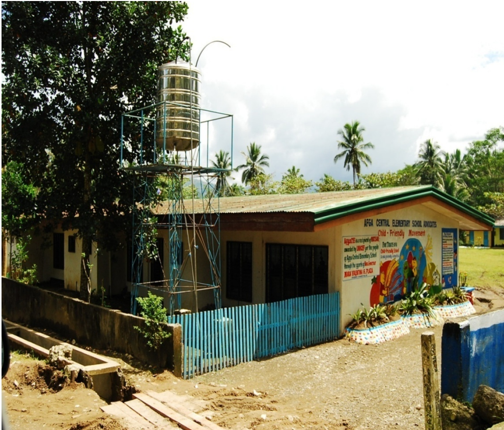
In April 2007, UNICEF constructed a water distribution system in Afga Elementary School. They built a 1,000-liter capacity elevated water tank to have a ready storage of water within the school premises. Photo by: Ida Marie Pantig.
