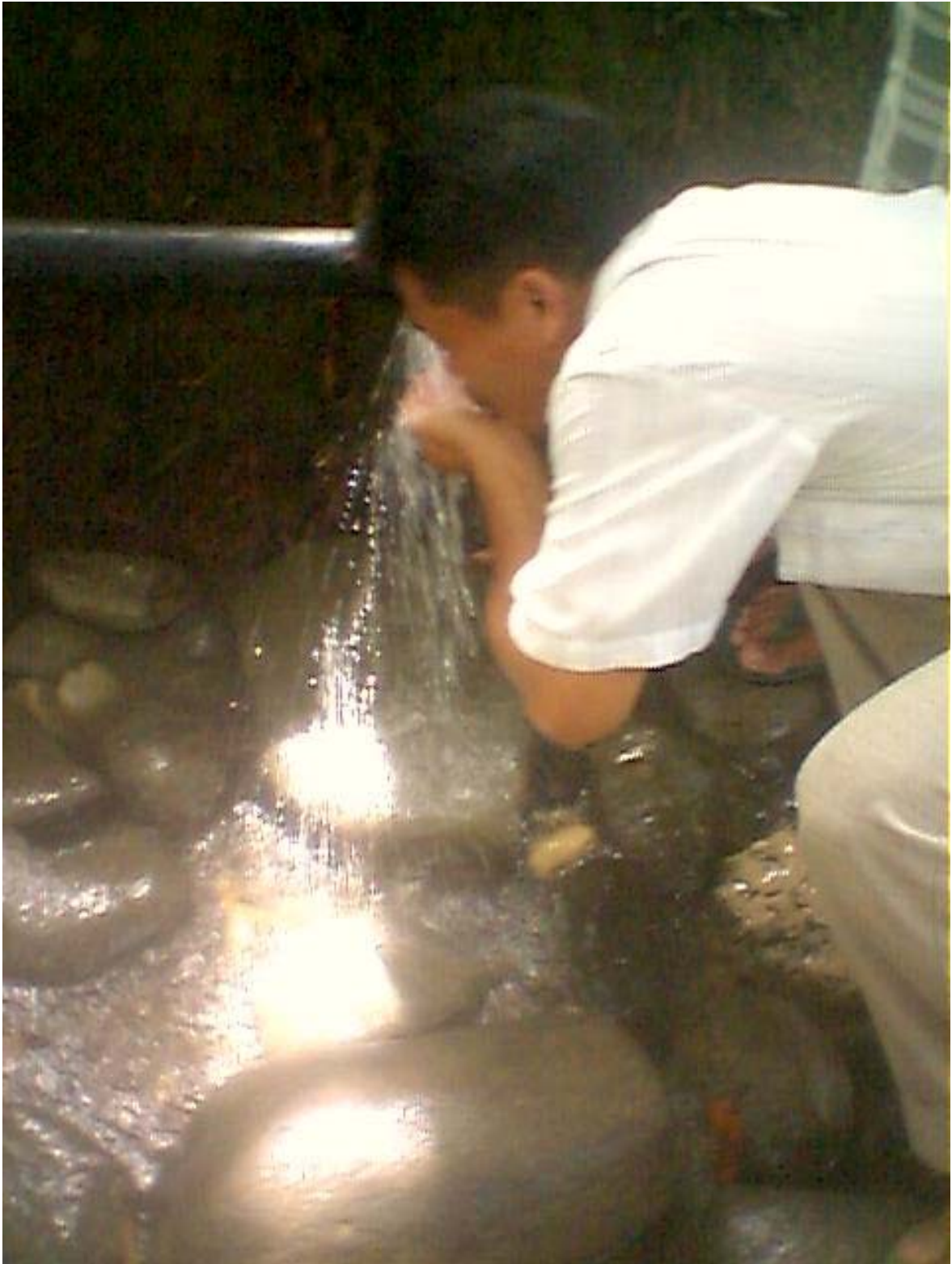
Level II Water System in Barangay Afga, Sibagat. Residents get their potable water through a pipeline connected to a communal water point (spring box). This is Barangay Afga's only potable water system. Photo by: Leilani Bolong.
