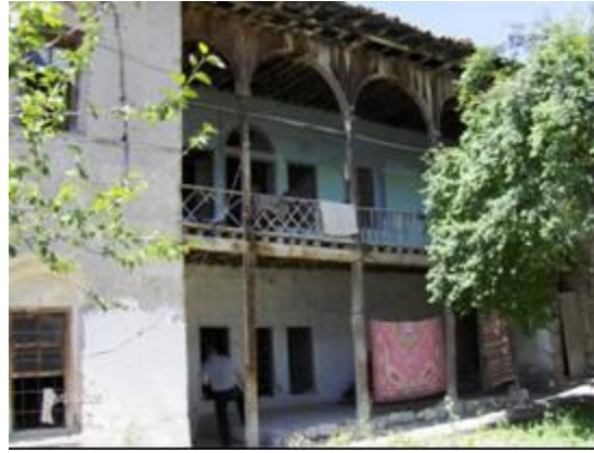
Figure 13. The courtyard of Poyrazlar House
