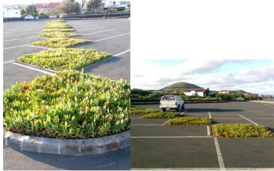
Figure 10: New parking facility decorated with one invasive specie.
