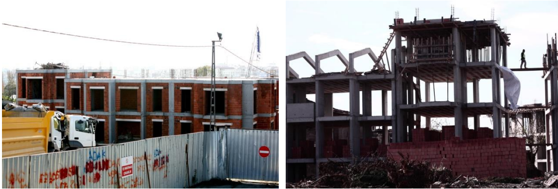
Photograph 2, 3: Construction of new and quotidian houses in Sulukule Photograph: Can Berkol, 25.11.2010
