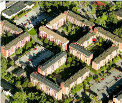
Fig .5 Husby, built during the mid 1970-ies. Higher blocks arranged around courtyards. Creating a more urban environment was a goal, which led to a rather dense built environment with higher buildings concentrated along the subway
