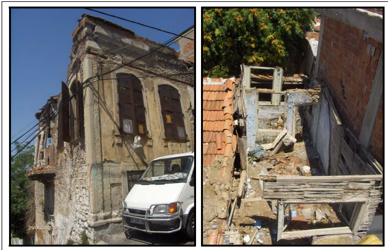
Photo 2: Ruined Historical Buildings
