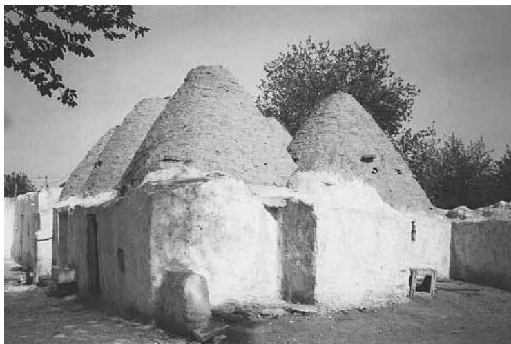
Photo 4 . Traditional Harran House
