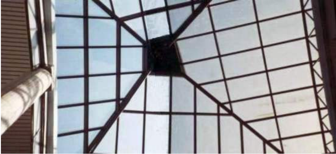
Photo 4: the new roof, invisible from the outside
