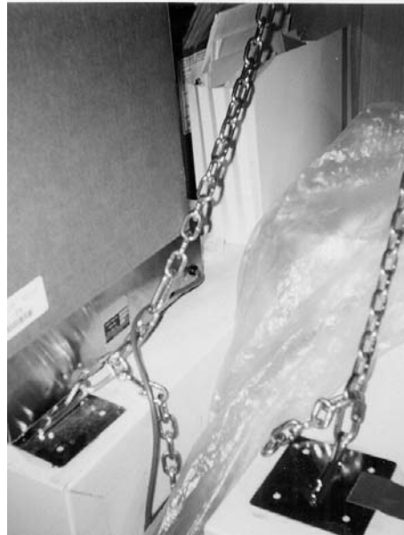
Figure B.2: Adhesive connections
