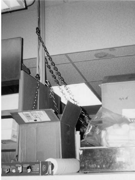
Figure B.3: Connection to strongbacks Figure B.4: Chain connection to wall
