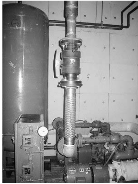
Figure A.2: Flexible piping connection
