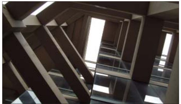
covered exterior lobby
