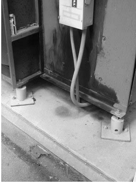
Figure A.3: Rooftop cabinet support
