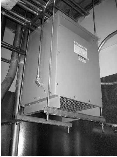
Figure A.11: Typical suspended cabinet Figure A.12: Typical strongbacks
