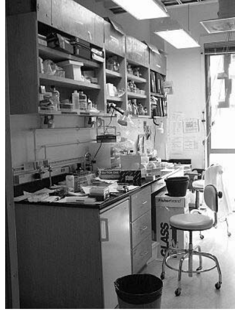
Figure B.10: Shelves with metal restraints (top)
