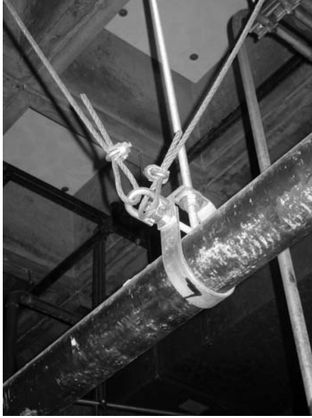
Figure A.1: Typical piping support
