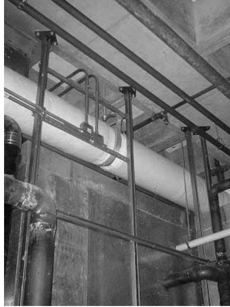
Figure A.11: Typical suspended cabinet Figure A.12: Typical strongbacks
