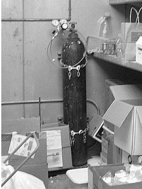
Figure B.5: Smaller tank restraint
