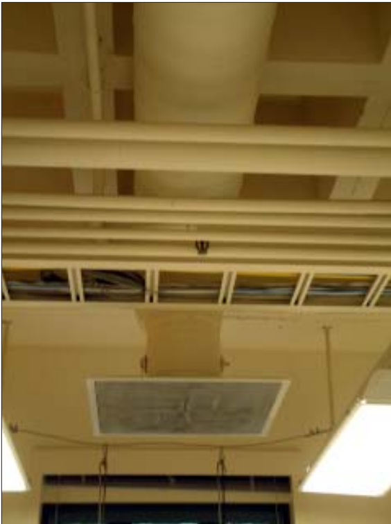
suspended air supply and cable tray
