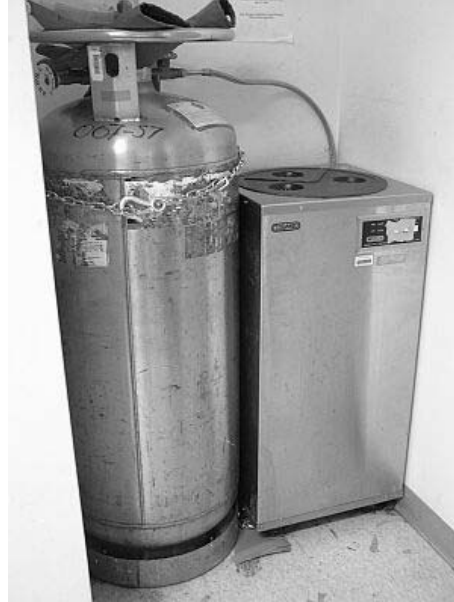
Figure B.6: Larger tank restraint
